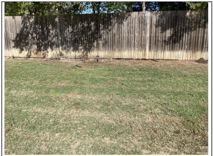
Sample of disconnected sprinkler line
