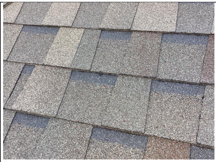
Sample of tread damaged
