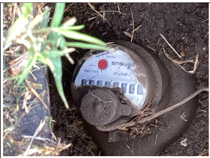
Photo of water meter showing no movement with all taps off
