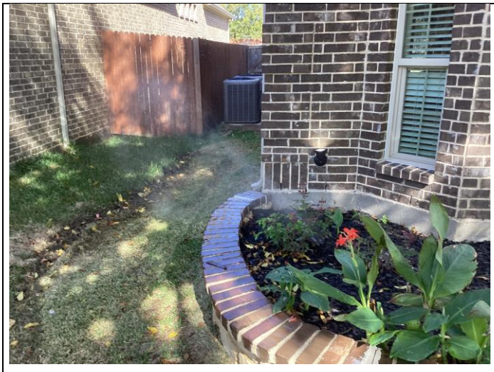
Sample of damaged drip line
